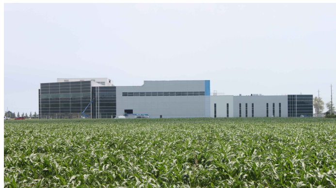
Darlington Energy Complex, Courtesy of Ontario Power Generation
